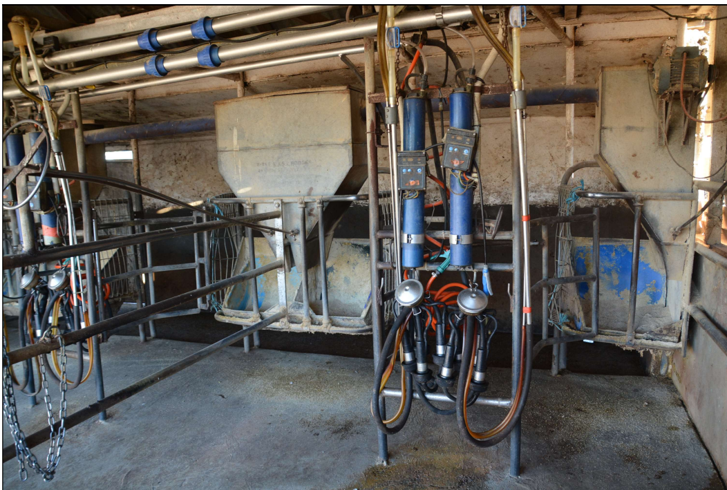
One of the milking bays and the milking machines. There will be one cow each side.
