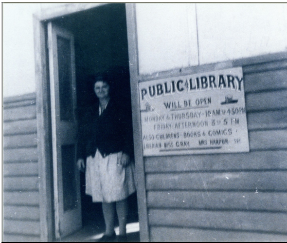
The doorway to the building. The years is unknown and the images comes from a copy negative from the Historical Society collection.
