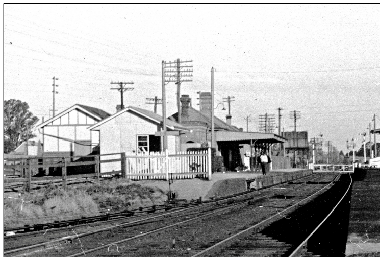
26 August 1939. Riverstone Railway Station. The building on the far left is the Ambulance Room viewed from the rear. Photo: Cropped from image ARHS 005586, Singleton CC Collection.
