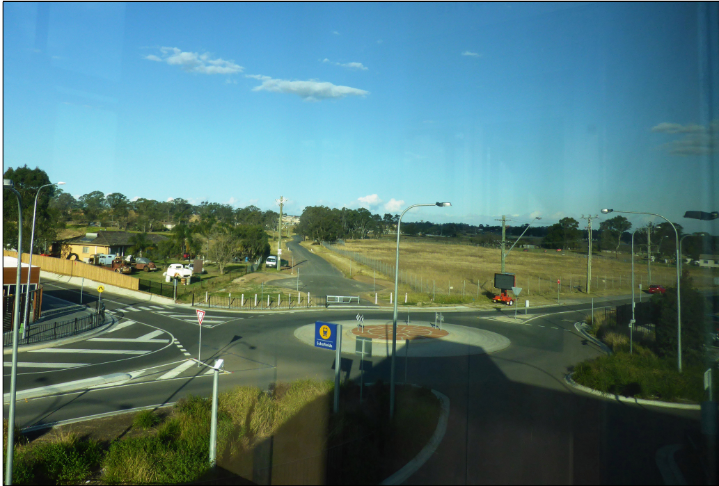
2 August 2014. Looking from the Schofields Railway Station to the future site of the Schofields Village. The roundabout was replaced by traffic lights in 2022. Photo: Rosemary Phillis.
