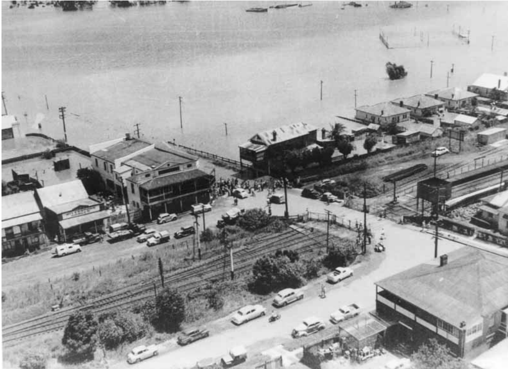
Aerial shot of Garfield Road over the railway line in the 1956 flood.
