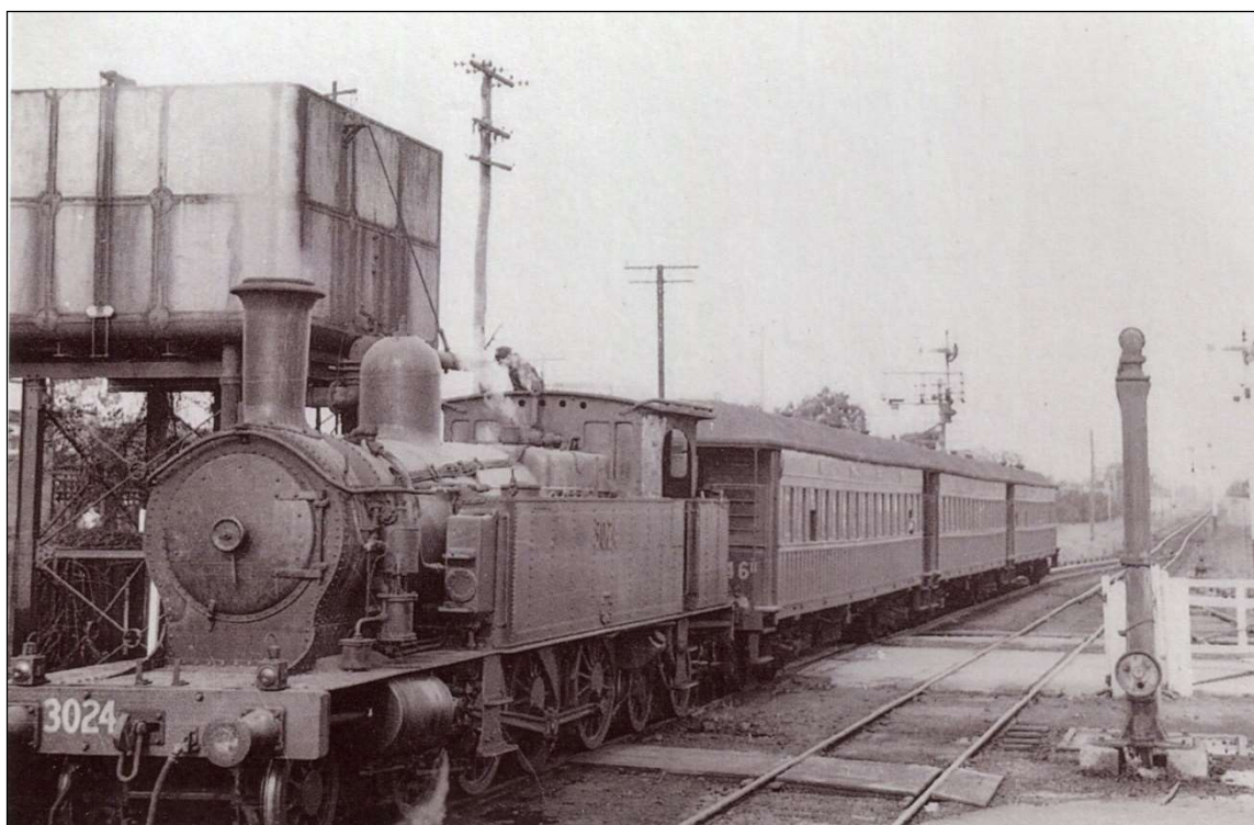
Riverstone Railway Station, 12 July 1958 Loco 3024 Regular Passenger Train
