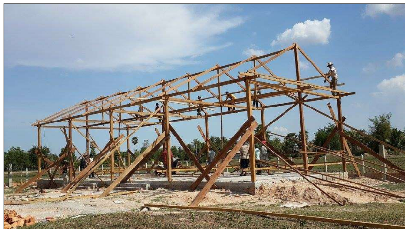
The school under construction.
